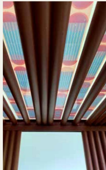
A set of stained-glass-style solar panels will be installed as part of the roof at the **DUTCH BIOTOPE PAVILION at EXPO 2020 DUBAI** (which has been moved to 2021 because of the coronavirus pandemic). Designed by **MARJAN VAN AUBEL**, the lightweight photovoltaics generate power while also letting tinted daylight through. Van Aubel created the colorful panels by using organic light-absorbing dyes that cover
